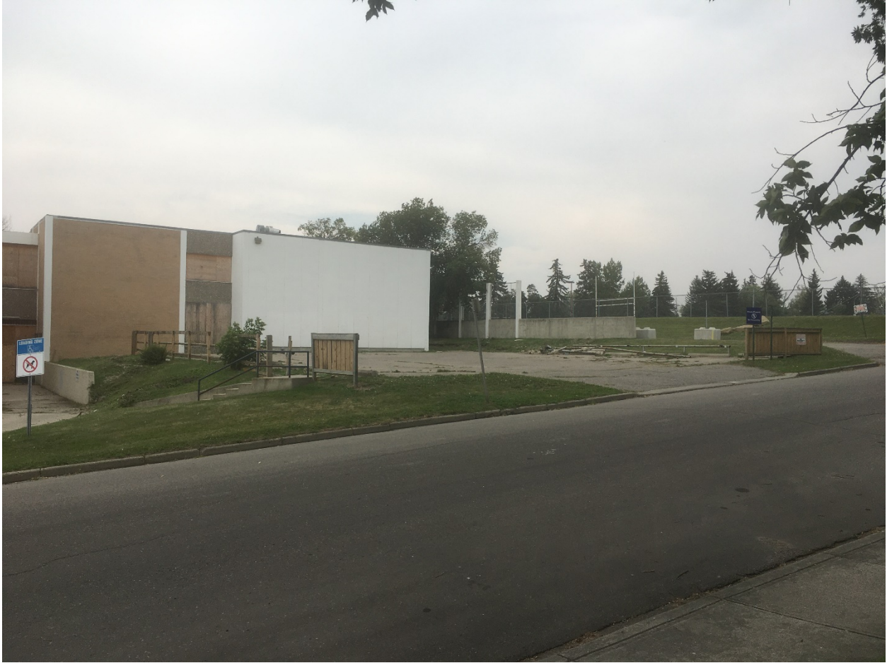
North-west site looking east
